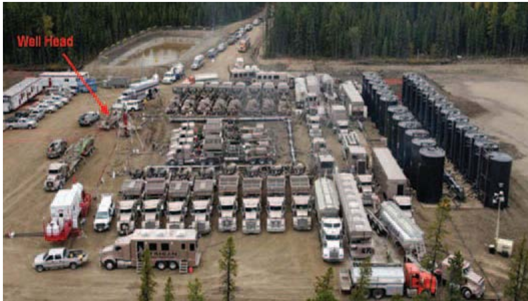
Figure 2. Infrastructure associated with shale gas well fracturing in the USA (from Warner 2011)
