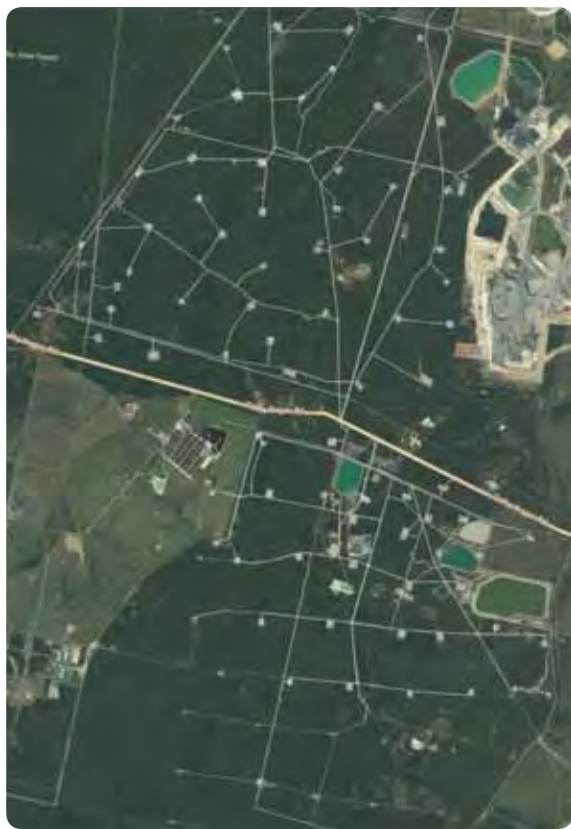
Figure 7.1: Aerial photograph showing the interconnected network of roads and other infrastructure in a CSG field near Dalby State Forest, Southern Queensland
