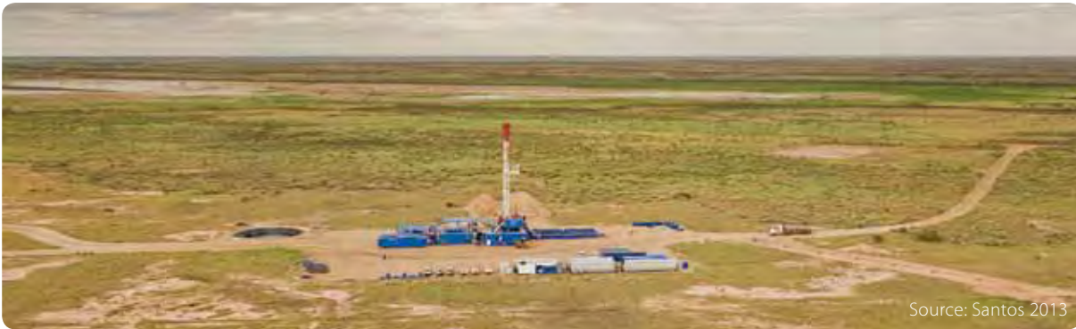
Figure 4.1: Well drilling in Australia
