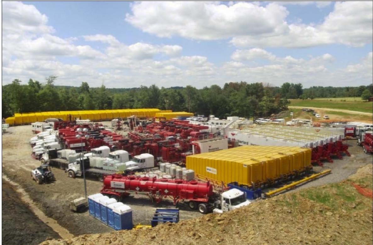
Figure 2.4 : Hydraulic fracturing, Marcellus Shale, West Virginia
