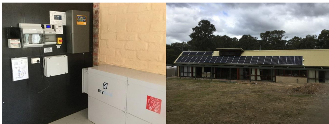
Figure 22 Jayne and Cathy's house with solar panels, inverter and battery system (Source: Jayne and Cathy)
